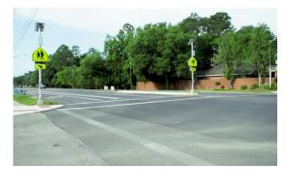
Tower Road and NW 43rd Street are two of Alachua County's most traveled roads. This year, both roadways received a major overhaul that included a complete resurfacing of both roadways, added crosswalks on NW 43rd Street and bus pullouts on Tower Road.
